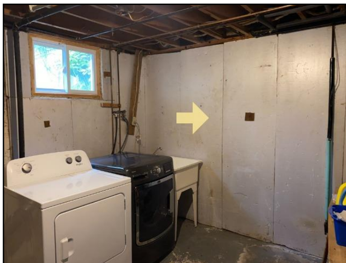
6. Exposed combustible insulation
